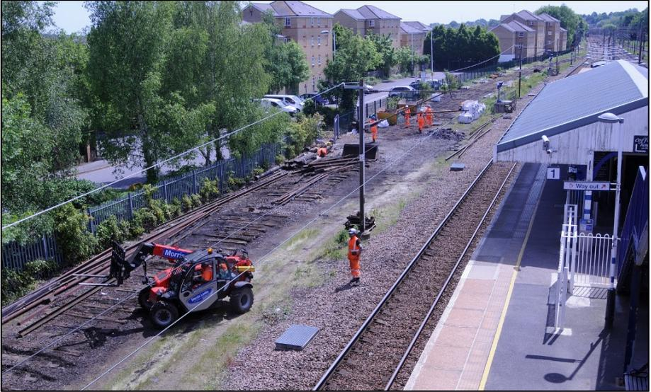
During May 2018 the 'up' siding at New Barnet was lifted, the track was in poor shape and only used for civil engineering road-railing plant etc. The siding is the last vestiges of the goods yard and shed that served the area. Possibly it may be re-laid as new materials are appearing ballast and such like, one to look out for.
