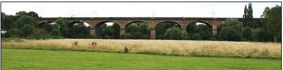
The **Wharncliffe Viaduct** crossed the valley and was brick-built at an elevation of 66 feet, built in 1836. The viaduct was the first major structural design by I K Brunel, It was also the first railway viaduct to be built with hollow piers.
