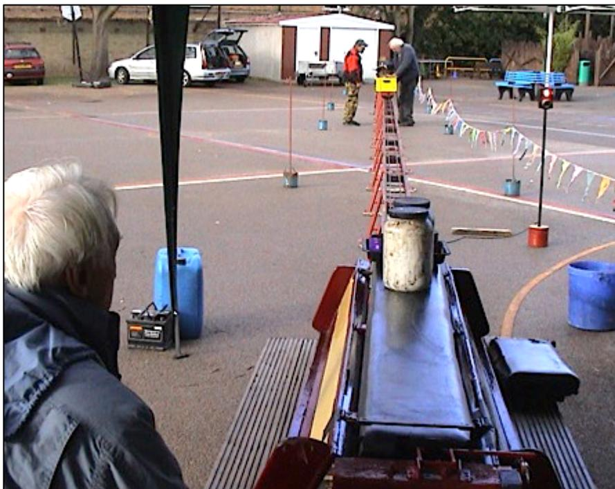
In the photo above the track has been set out across the school playground and Peter and Matt are 'walking the line' with a spirit level on a wagon to check for horizontal alignment of the railhead prior to the opening of the event. Much care is given to the levelling and straightness of the track to ensure comfortable and safe operation of the trains.
