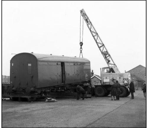
*Sleepers were used to support the van between lifts.*
