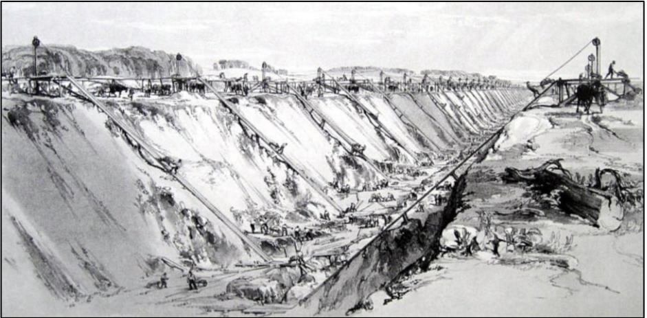
the cutting forty feet deep and up to sixty feet deep on a section of about half a mile. That was some achievement when the chalk had to be mainly dug by hand with horse whips to take the barrows up on boards to the top for disposal. Remember that this was the era of stage coaches and before the development of drag lines and mechanical excavators.
