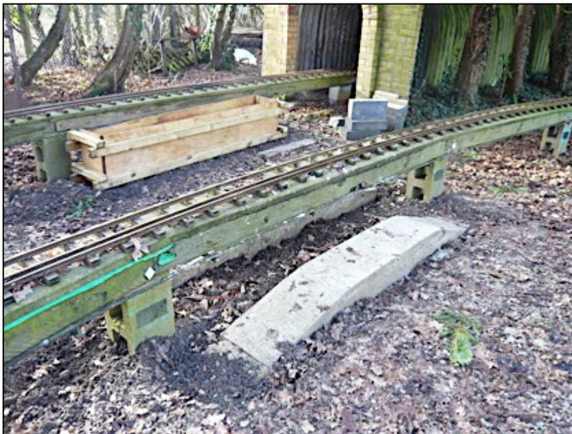
**The Raised Track is now closed until further notice**, whilst we make and pour concrete into the shuttering to make the four step-over blocks to assist access to the tunnel shed and the COSH cabinet.
