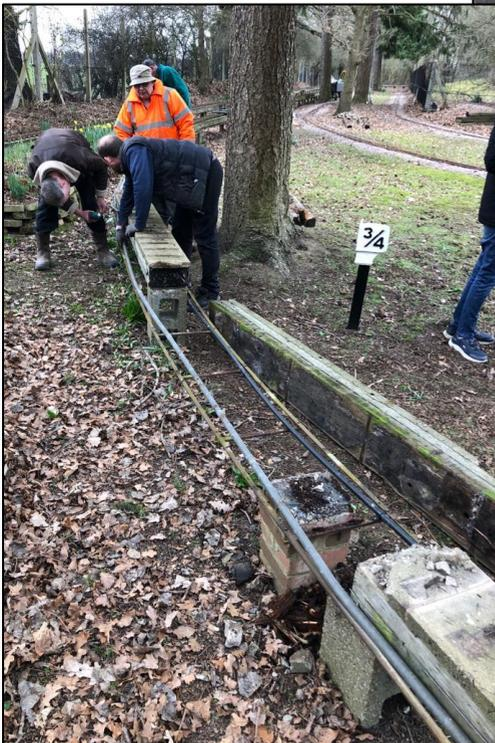
The club carries a small stock of serviceable sleepers for just this eventuality. As you can see from the pictures once the sleeper was removed all that remained were the anti-ti-p rails and signalling conduit
