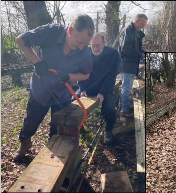
Sections of the track had to be removed. New sleepers were cut to size and placed onto the concrete piers.
