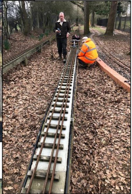
The job is now well advanced. and a new concrete screed laid (see front page) before the track could be installed.
