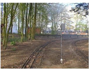
The Narrows exit signal with the 'Not in use' board **Photo:** Alan Marshall
