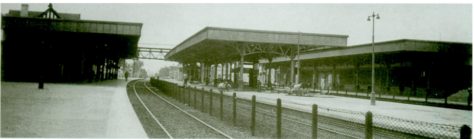
8. Buenos Aires Great Southern Railway: Louras de Zamora suburban station 9.5 miles from Buenos Aires, Plaza Constitución terminus, looking south about 1926. Note the wire fence between the tracks to stop passengers alighting on the wrong side.
