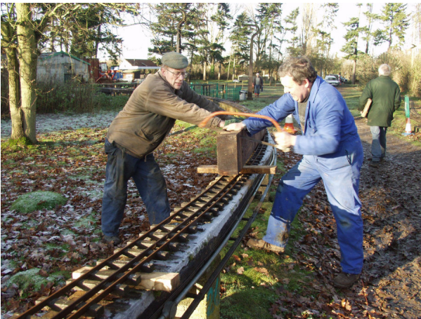
Left: A few of the timber sleepers that form the structure of the raised track have reached the end of their useful life. Mike Foreman (left) and Grahame Gardner have been replacing them.
