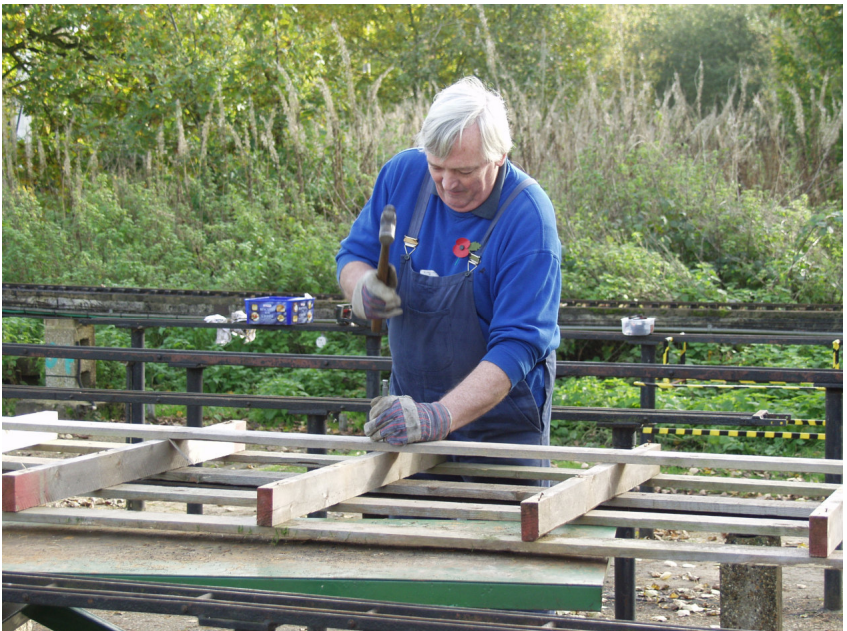
Some innocent piece of shuttering gets a hammering from Peter Davies
