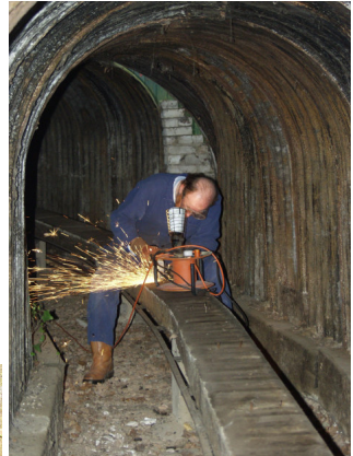
Left: A few of the timber sleepers that form the structure of the raised track have reached the end of their useful life. Mike Foreman (left) and Grahame Gardner have been replacing them.
