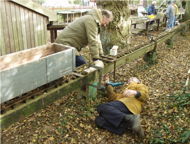
Right: With the old track removed from the tunnel, its securing pins had to be cut off before the new track sections could be positioned. Mick Avery used an off-hand grinder in the gloom for this task.
