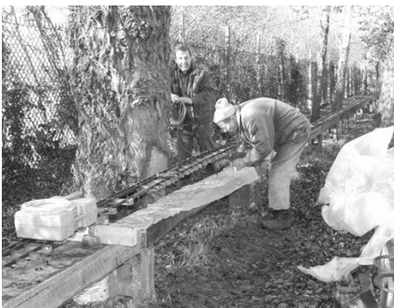
Routine maintenance of the raised track involves replacing decayed structural sleepers.
